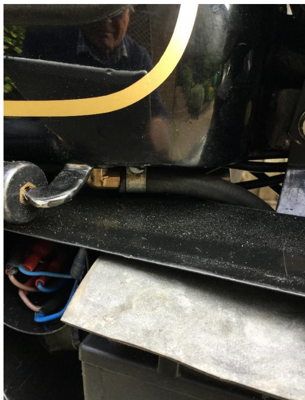
Right angle bend replacing petrol tap
